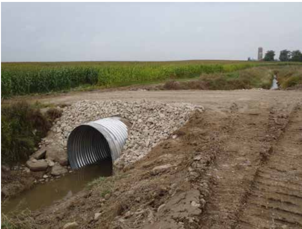
Figure B1–1. Rural drainage works.
