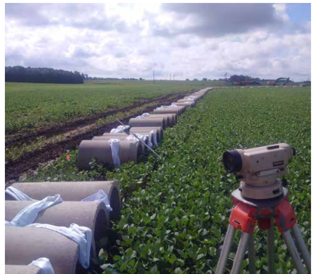
Figure B10–12. Concrete pipe (with geotextile) prior to installation.
