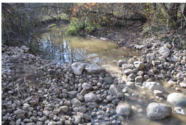
Figure B11-5. Newbury weir.
