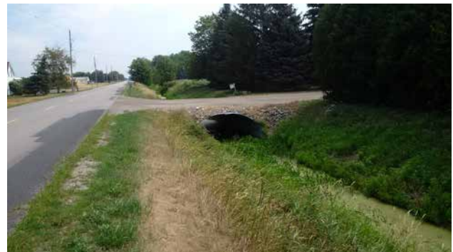
Figure B10–1. An open-bottom crossing/pipe arch.
