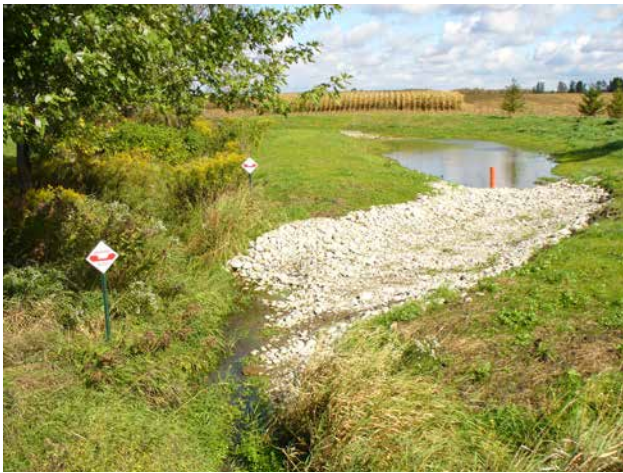
Figure B7-2. An off-line sediment trap.
