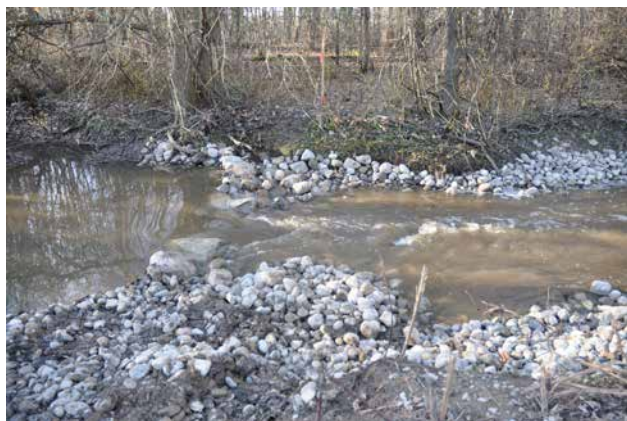
Figure B3–6. A Newbury weir.
