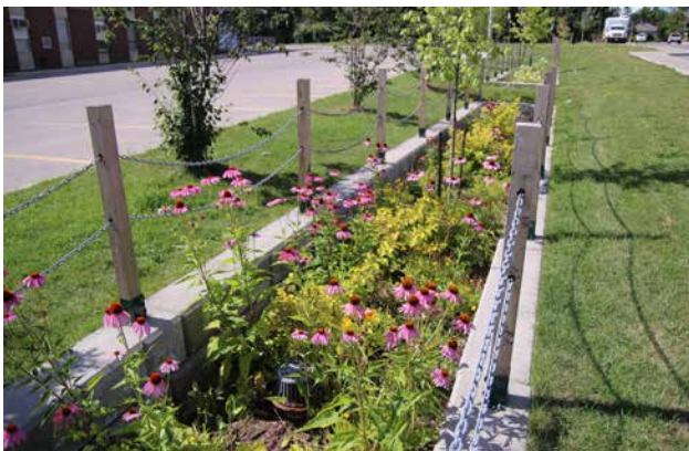
Figure B5–1. A bioswale is an example of a LID technique used to reduce surface water runoff.
