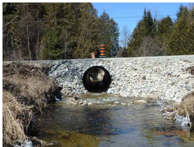
Figure C9–4. A large-diameter culvert on a non-listed waterway.
