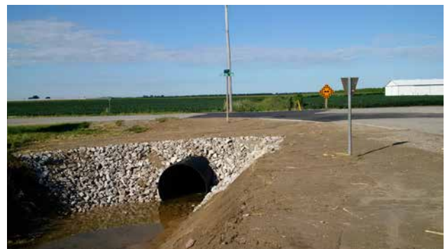
Figure B10–2. An embedded culvert.
