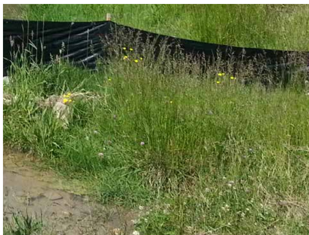
Figure B6–3. A silt fence installed next to a drain.
