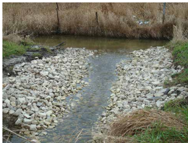
Figure B7-5. Riprap armouring of a drain.
