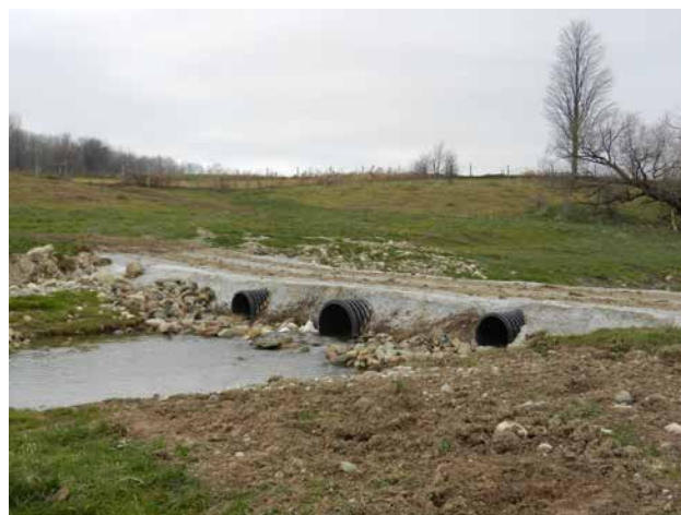
Figure B3–7. A low level crossing.
