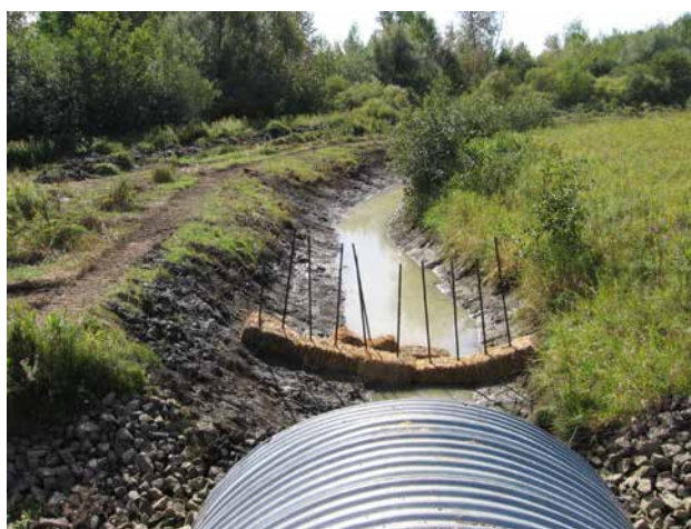
Figure B6–2. A straw bale check dam.
