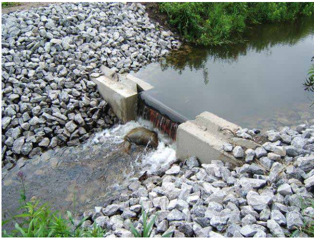
Figure B10-27. A small dam.
