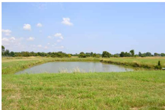
Figure B10-24. A wet pond always contains water.
