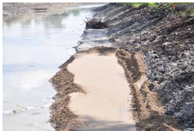
Figure B11-6. A dewatered channel with gravel substrates on a littoral shelf.
