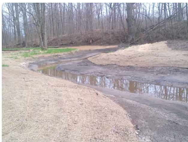
Figure B7-4. Rolled erosion control product installed on the banks of a drain.
