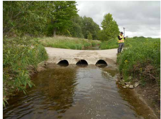
Figure B10-8. A low-flow crossing.
