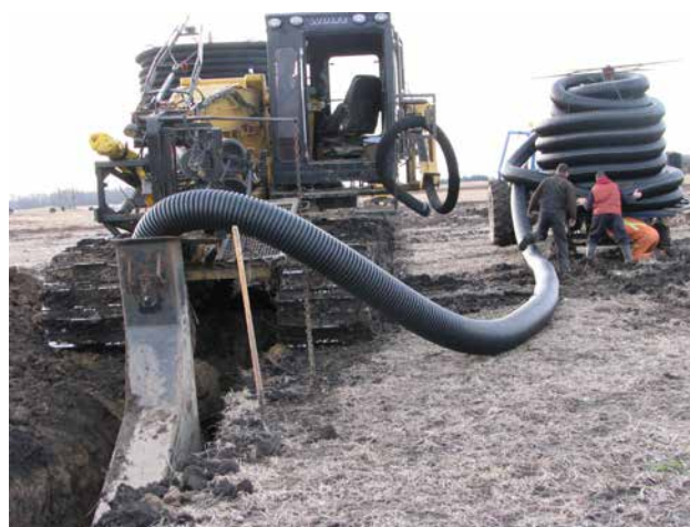
Figure B3–1. A contractor installing a rural piped drain.
