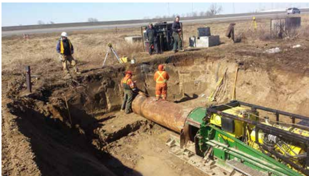
Figure B10–5. A trenchless crossing.
