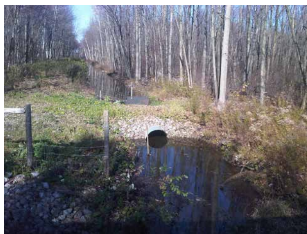
Figure B8–2. A wetland drain restoration project.
