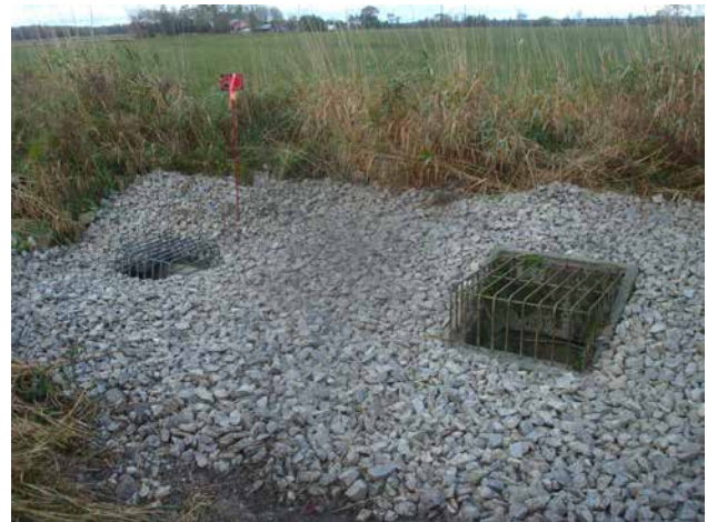
Figure B10–19. Birdcage grate with stone apron.
