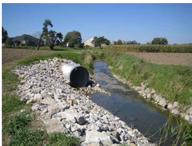
Figure B2–2. Example of a good outlet.
