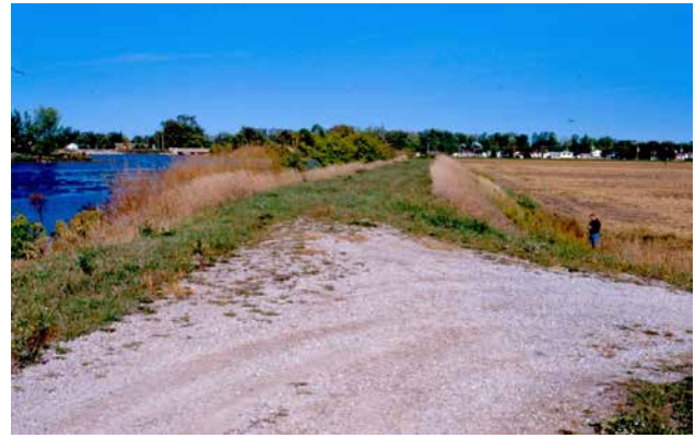
Figure B10-29. A dyke used to keep water out of the adjacent low-lying land.
