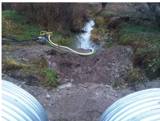
Figure C3–1. Dewatering for a culvert installation.
