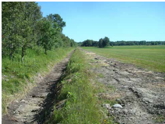
Figure B10–30. Excavated material spread to the right of the drain on farmland.
